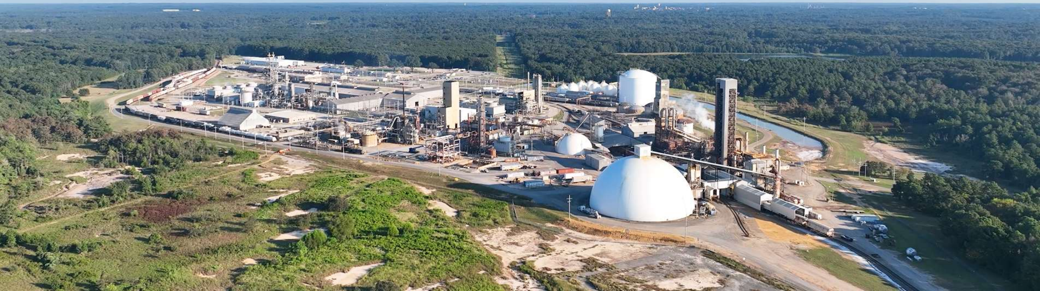
LSB Industries – EL Dorado Chemical Plant
